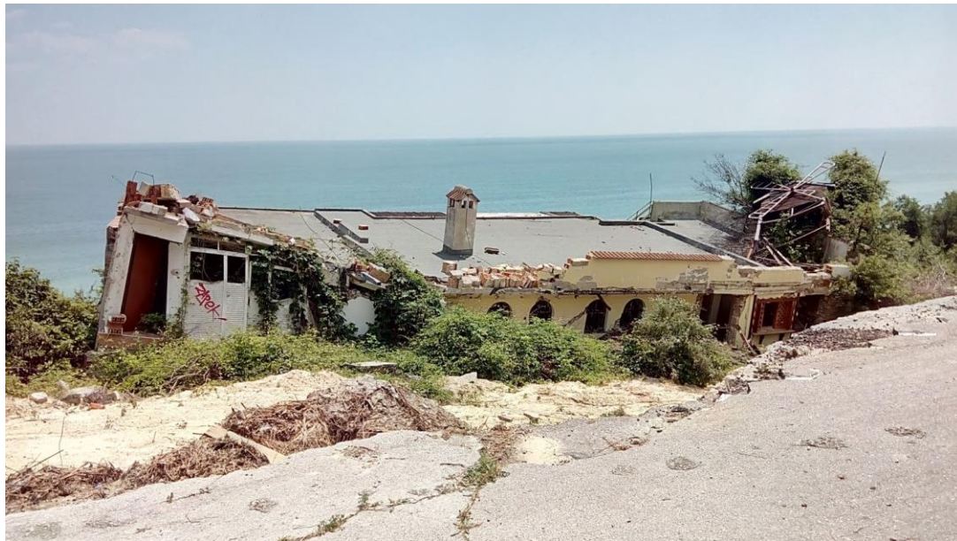
The landslide area “Trifon Zarezan Lanslide”, resort Golden Sands
